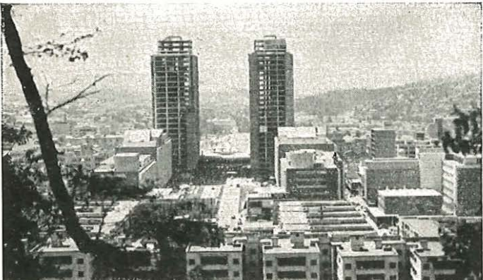
VENEZUELA BIC Construction Co. have undertaken the jointing and supervision of installation of a 448 pair 20 lb trunk cable to improve the telephone service between Caracas and Maiquetia. With a route length of approximately seventeen miles, the cable runs wholly in ducts along the side of a newly-constructed auto-road linking the capital town of Caracas with the coast. This contract has been undertaken for the Compañia Anonima Nacional Telefonos de Venezuela, the cable being manufactured by BICC.
