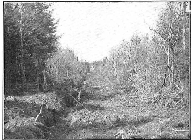
FIG. 5.—RIGHT OF WAY CLEARED BETWEEN ADEYTON AND HILL VIEW.
