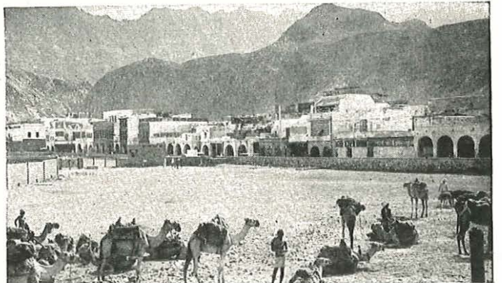
ADEN To extend existing facilities and to cater for the Colony's growth, a new distribution network has been installed comprising approximately 44 miles of BICC cables specially protected against soil corrosion. The new network provides an increase of 3,000 lines and consists of cables of varying sizes ranging from 15 to 200 pairs, twin cables, the larger sizes being of the unit twin type. A short balanced and loaded trunk cable was also installed to link the Town with the new refinery site at Little Aden. This contract was undertaken for the Aden Posts and Telegraph Department.
