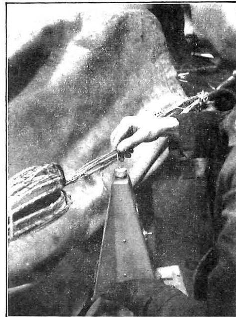
FIG. 9.—SOLDERING ALUMINIUM CONDUCTORS TO COPPER CONDUCTORS.
