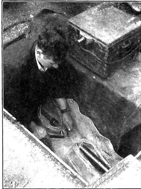
FIG. 6.—WELDING A JOINT IN THE ALUMINIUM CONDUCTORS.
