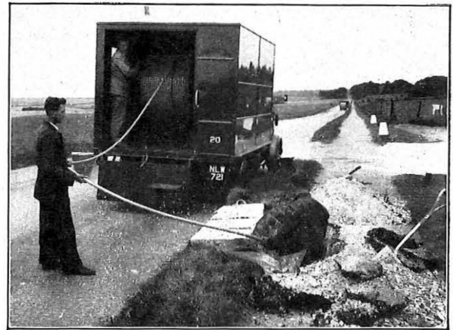
FIG. 3.—DRAWING-IN THE CABLE.
