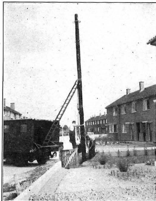
ERECTING A POLE WITH THE DERRICK.
