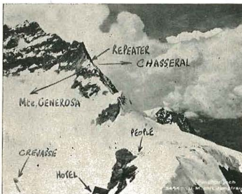
This view was sent to G.E.C. by the Company's installer, and illustrates the difficulty of establishing the relay station at 12,000 ft. on the Jungfrauoch.
