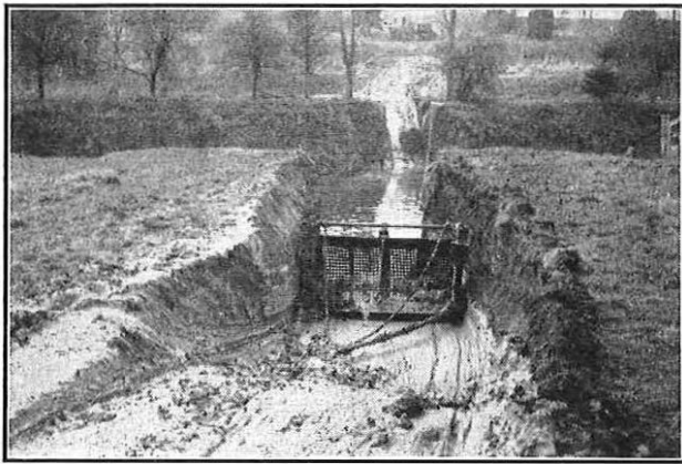
DREDGING THE CHANNEL ACROSS RIVER AVON.
