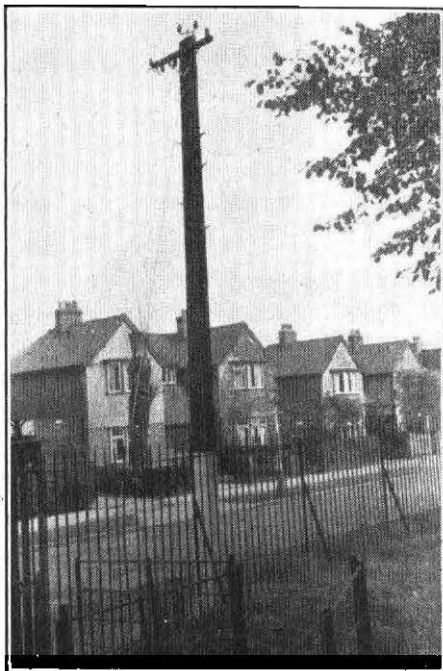
"HALVED" POLE ERECTED.
