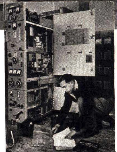
A member of the New Zealand P. T. & T. staff making adjustments during installation.
