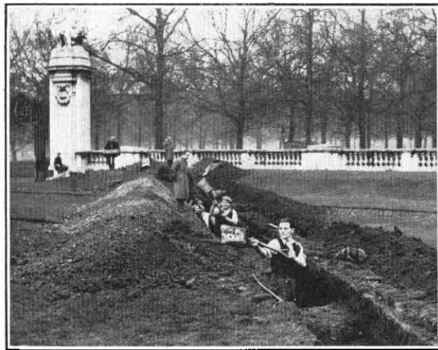
FIG. 2.—EXCAVATING FOR DUCT ROUTE NEAR CANADA GATE.
