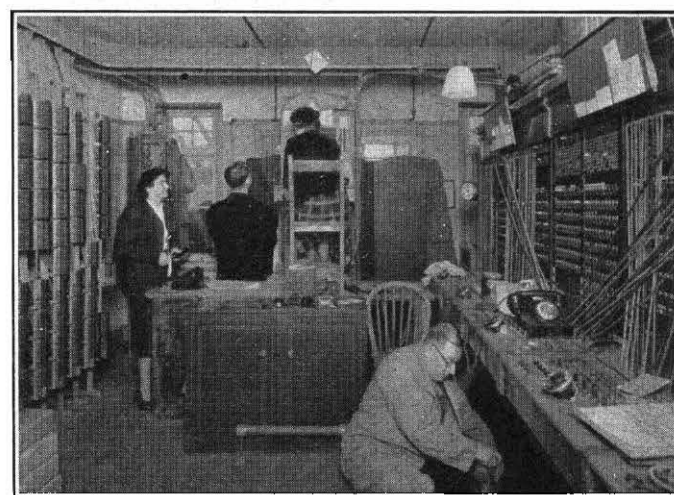
P.B.X. 10 + 50 MOUNTED ON PLATFORM IN CANVEY EXCHANGE.
