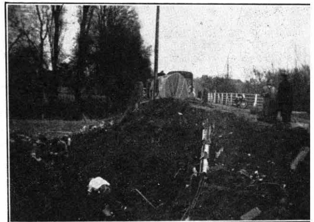
CABLE REPAIRS IN PROGRESS.
