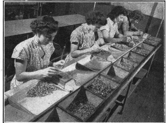
FIG. 4.—SOLDBRING WIRES TO BRIMISTORS.
