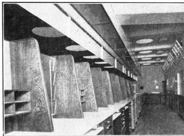
THE COUNTER LIGHTING INSTALLATION.
