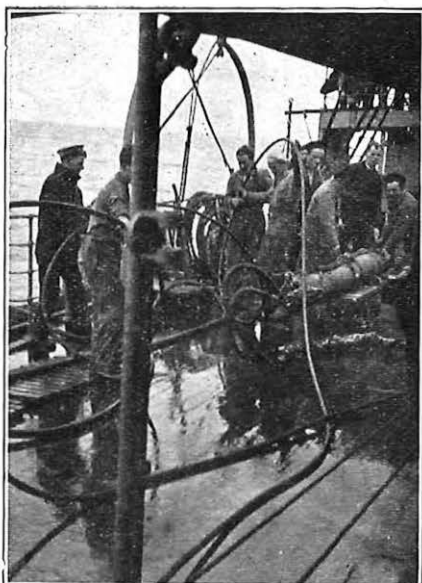
TAKING TURNS OFF AFTER CABLE DRUM TO PASS THE REPEATER AFT.
