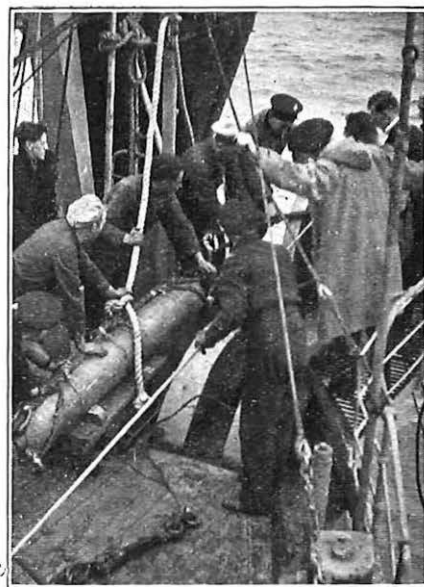
THE REPEATER AT THE STERN SHEAVE.
