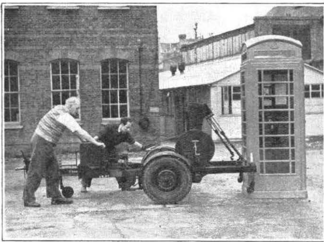
FIG. 1.—PLACING TRAILER AROUND KIOSK.
