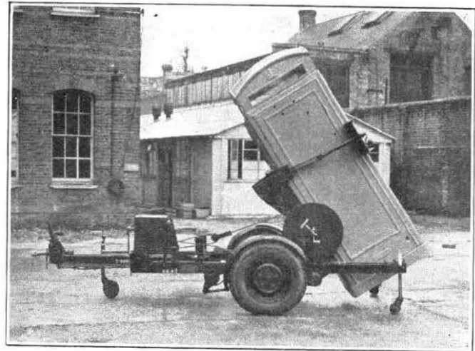
FIG. 2.—KIOSK LIFTED AND BEING TURNED.
