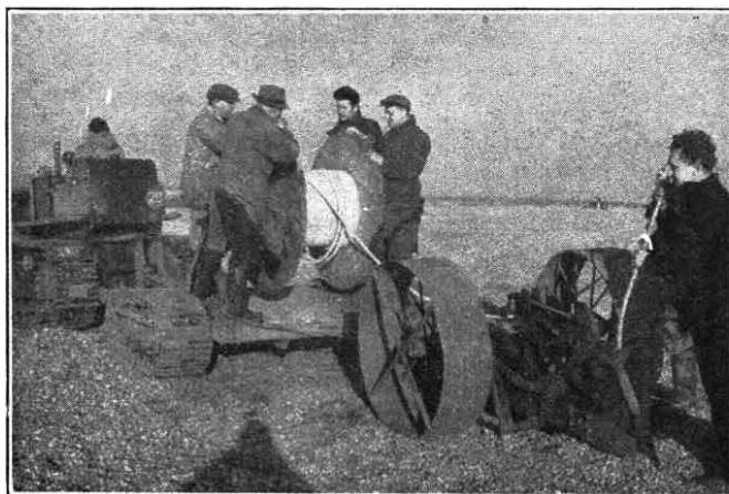
MOLEDRAINING CABLE IN SHINGLE.
