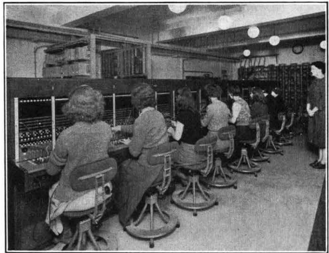
FIG. 3.—THE ADMINISTRATION SWITCHBOARD.
