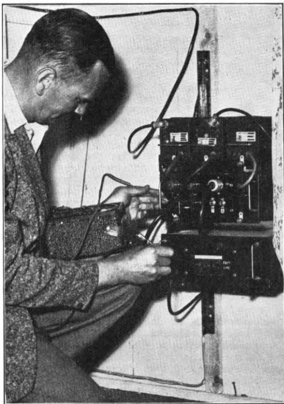
THE TRANSMITTER AND RECEIVER UNIT AT HERM.
