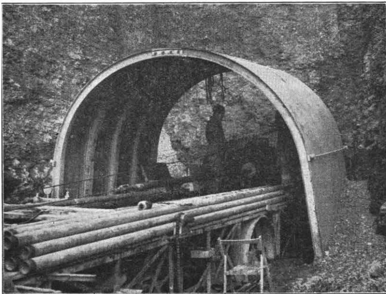
FIG. 8.—DRILLING RIG AT ENTRANCE TO LATERAL BOREHOLE.
