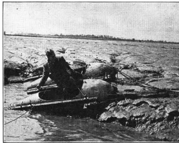
CROSSING A SMALL CREEK. CABLE CAN BE SEEN ENTERING TUBE BELOW DRIVER'S RIGHT ARM.
