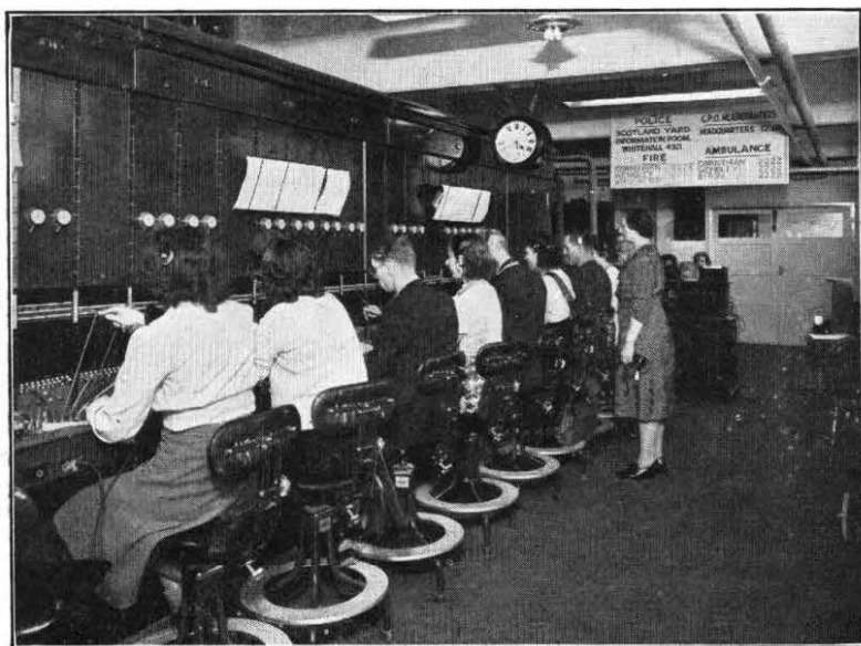
FIG. 1.—CORINTHIAN EXCHANGE—PART OF SWITCHBOARD
