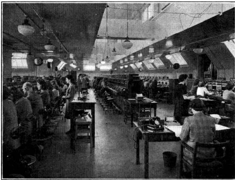
FIG. 3.—GENERAL VIEW OF THE SWITCHROOM.
