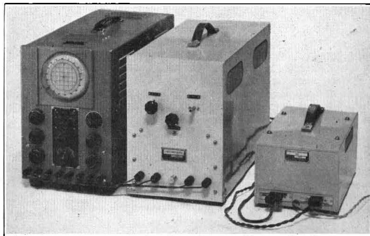
FIG. 2.—CABLE FAULT LOCATOR.
