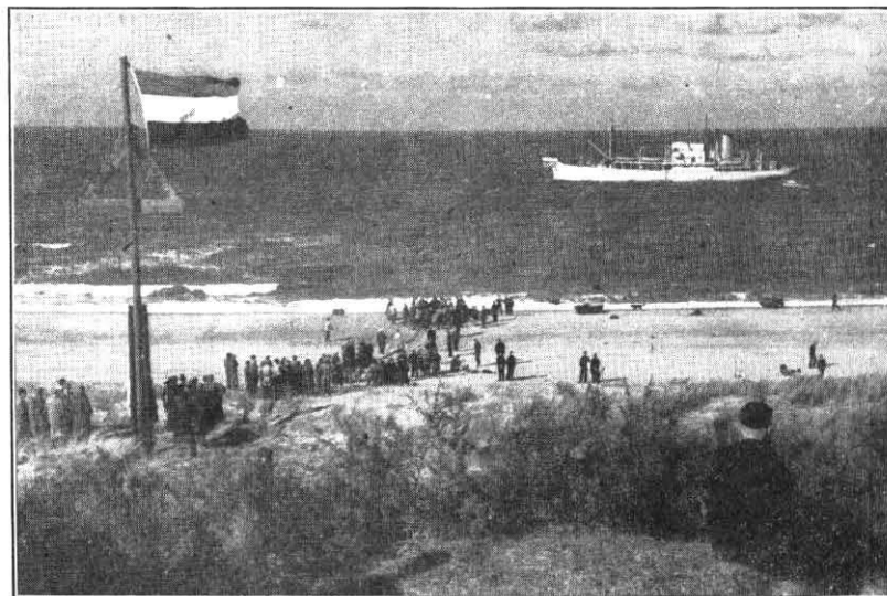
FIG. 4.—H.M.T.S. Albatross LAYING SHORE END AT DOMBURG.
