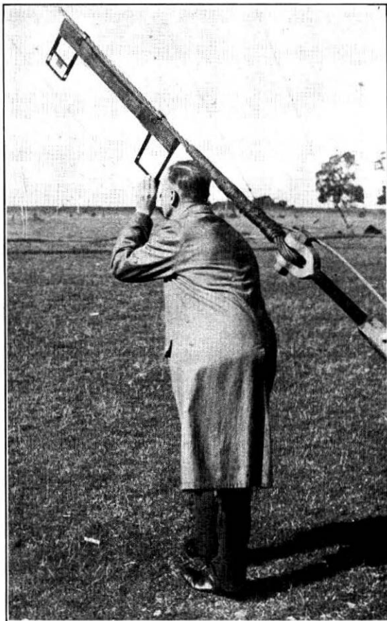
FIG. 4.—STAY-SIGHTING DEVICE.
