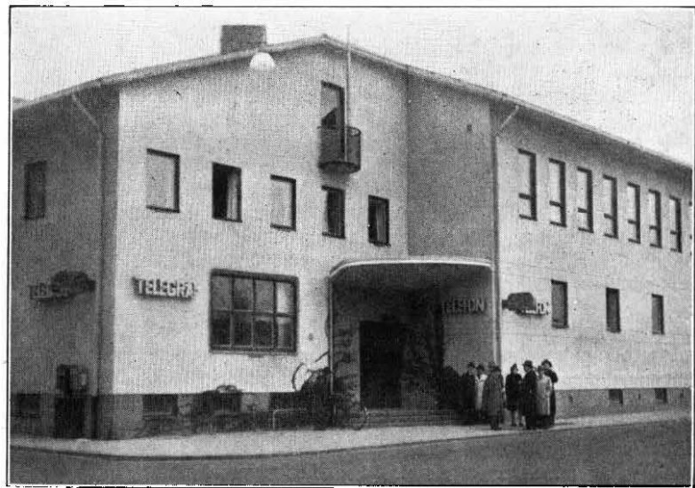
FIG. 2.—TELEGRAPH AND TELEPHONE BUILDING IN KRISTIANSTAD.
