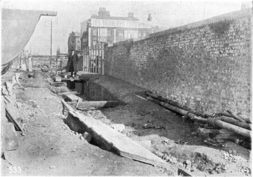
12.—SOUTH SIDE. SHOWS PIPES BEING CONCRETED IN.
