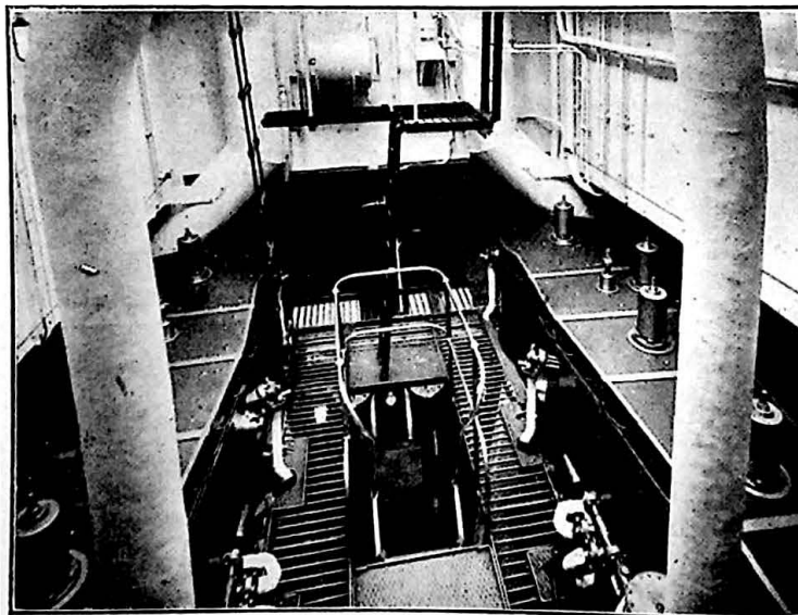
FIG. 6.—H.M.T.S. "IRIS." ENGINE ROOM (LOOKING AFT).
