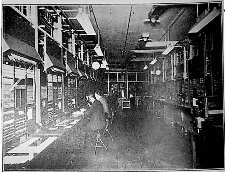
FIG. 3.—TRUNK TEST RACKS IN CITADEL.
