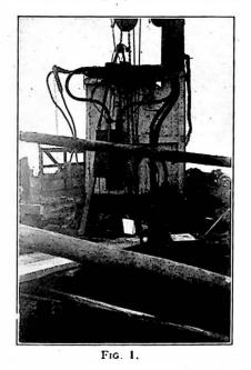
of the cable. They were then lowered into the manhole excavation, and positioned on a prepared reinforced concrete base, after which the manhole was built around them.
