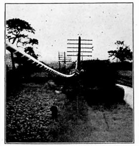
FIG. 4. CABLE SPAN PARTLY COMPLETED.
