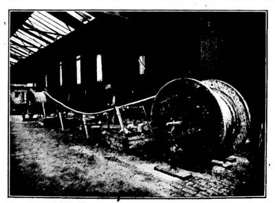
FIG. 1.-CABLE IN POSITION FOR RECONDITIONING.
