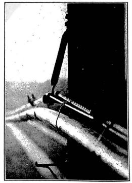
FIG. 5.—CABLE SUPPORTED BY MAIN AND AUXILIARY SUSPENSION WIRES.
