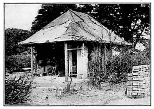
reinstated and the local builder proceeded with the work that same hour. Being unable to obtain Moler blocks for inside walls a local absorbent "white" brick was used and one window aperture bricked up pending cessation of the war. To obtain ventilation and occasional natural light it was also decided to dispense with glazing in the other window and fix wooden "panes" instead.
