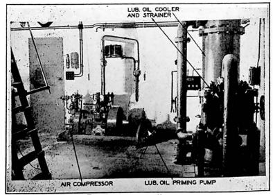
FIG. 5. AUXILIARY EQUIPMENT.
