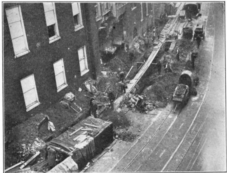
FIG. 6. BRIDGE CARRYING INTERRUPTION CABLE OVER BOMB CRATER.
