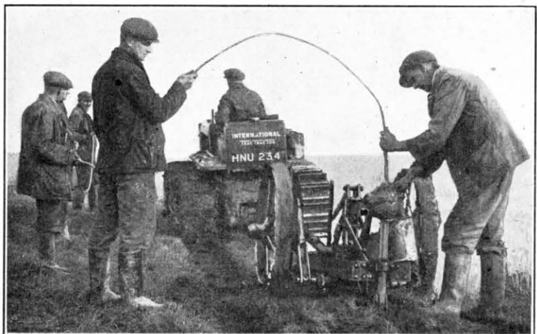
FIG. 2.—CABLE-LAYING WITH MOLEDRAINER.
