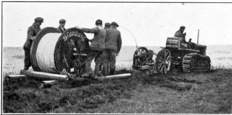
FIG. 3.—CABLE-LAYING WITH MOLEDRAINER AND SLEDGE.
