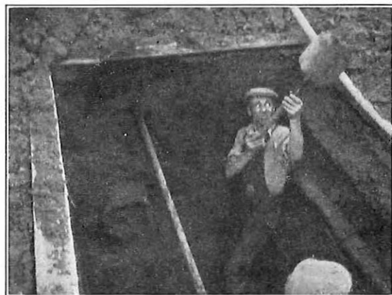
FIG. 5.—MANHOLE EXCAVATION IN WET SITUATION.
