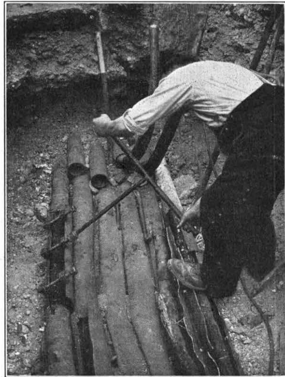
FIG. 4.—USE OF THE SCREW CLAWS.
