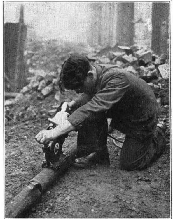
FIG. 2.—"SKILSAW" CUTTING STEEL PIPE.
