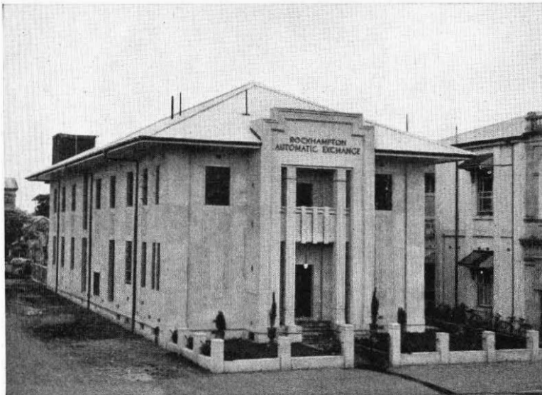
This exterior view shows the modern two-story building in which the equipment is installed.
