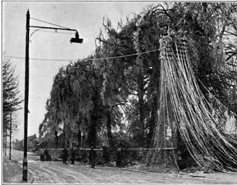
FIG. 7.—DAMAGE IN THE BRISTOL AREA.
