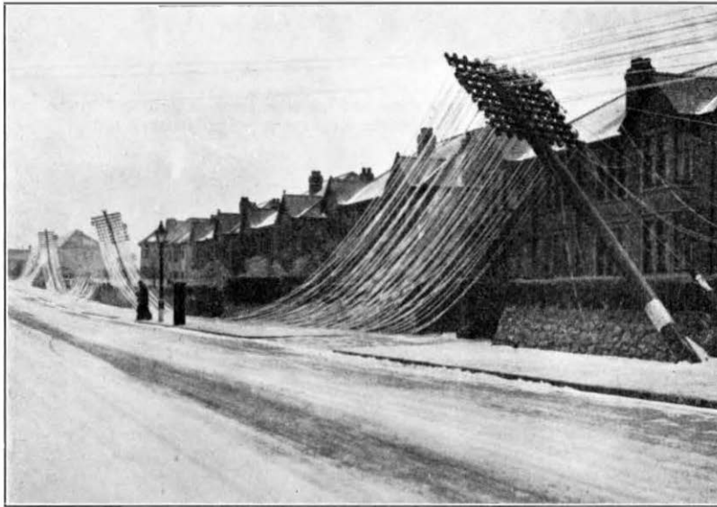
FIG. 3.—DEFLECTED POLES AT CYNCOED, CARDIFF.
