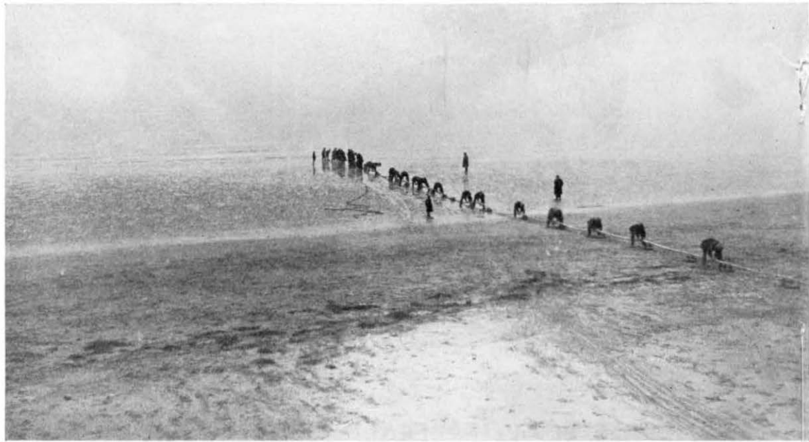
LAYING SUBMARINE TELEPHONE
