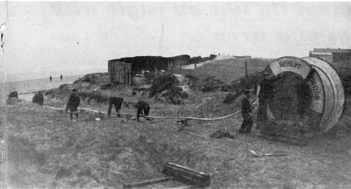
THE CABLE ACROSS AN ESTUARY
