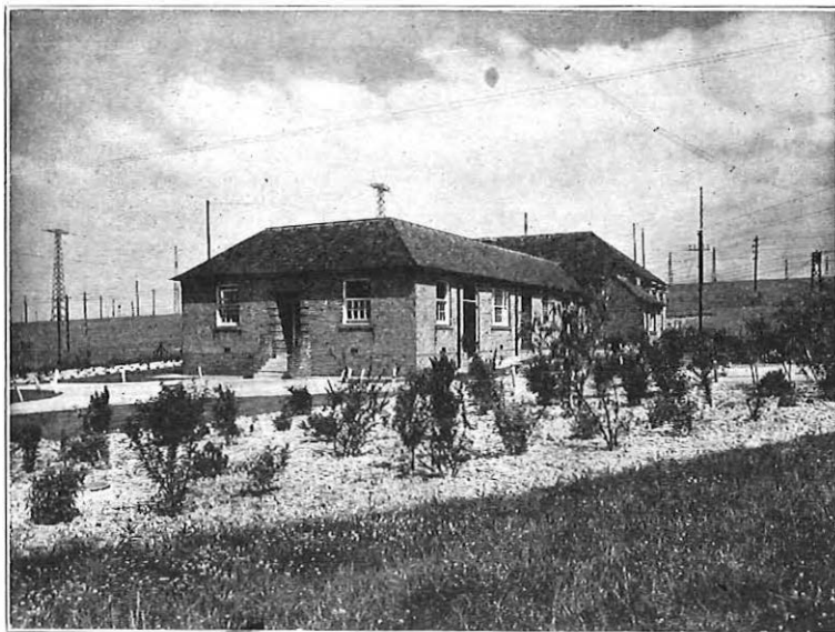
FIG. 1.—BALDOCK RADIO-TELEPHONE RECEIVING STATION.
