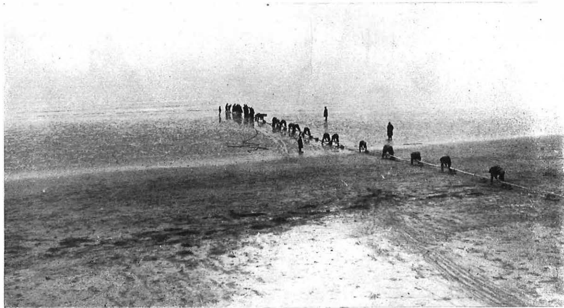
LAYING SUBMARINE TELEPHONE CABLES
