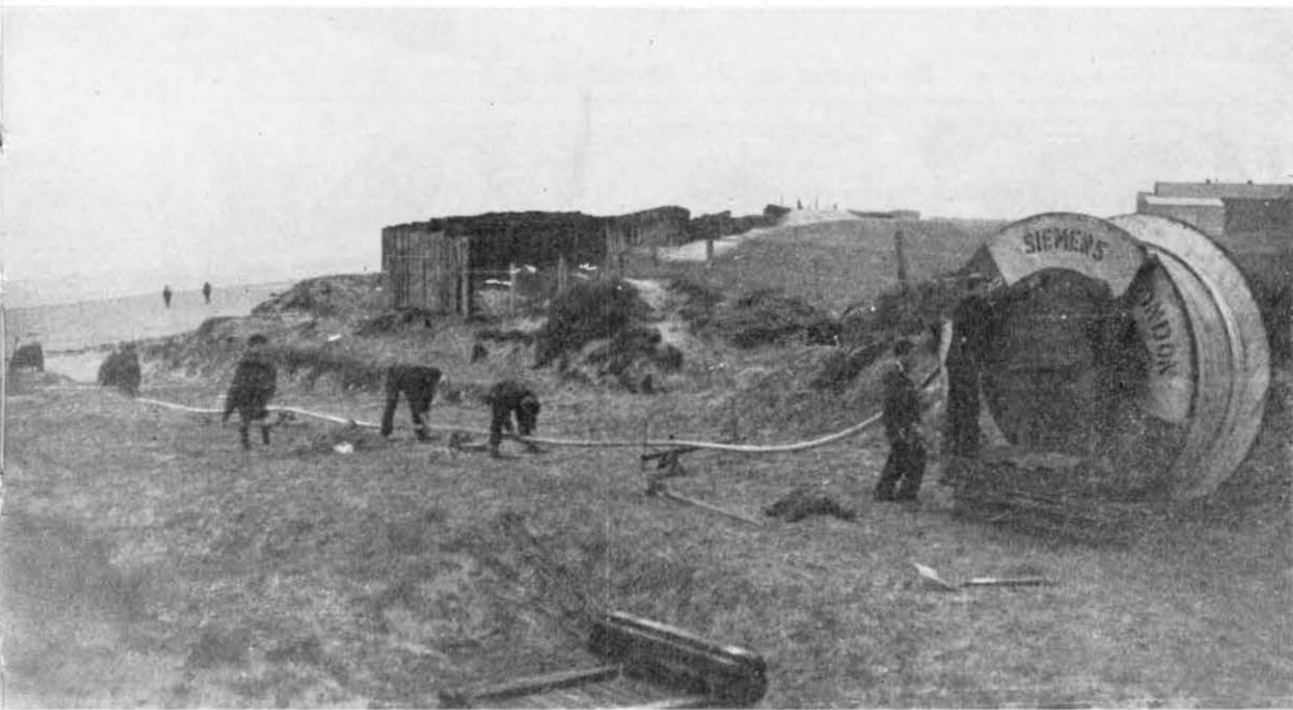
E CABLE ACROSS AN ESTUARY
