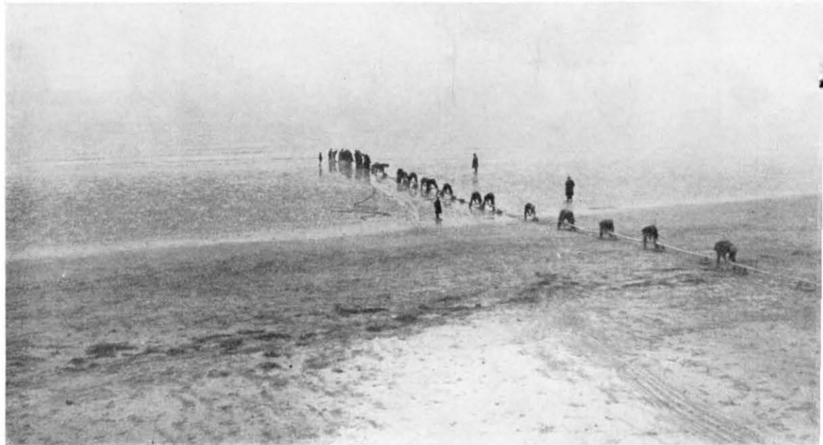
LAYING SUBMARINE TELEPHONE CABLES
