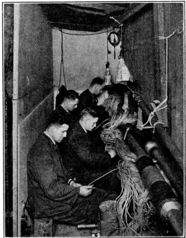
FIG. 11.—JOINTING WORK IN PROGRESS.
