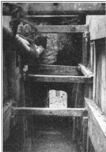
FIG. 3.—TUNNELLING UNDER SEA WALL.
