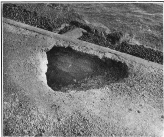
FIG. 1.—FOOTWAY SUBSIDENCE.
