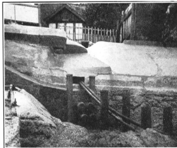
FIG. 4.—NEW PIPES IN POSITION.
