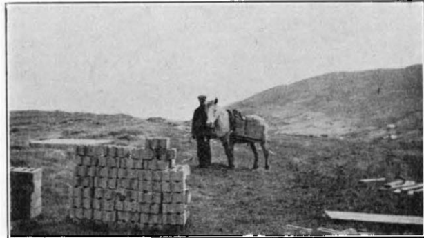
FIG. 1.—HORSES CARRYING BRICKS TO SITE.
