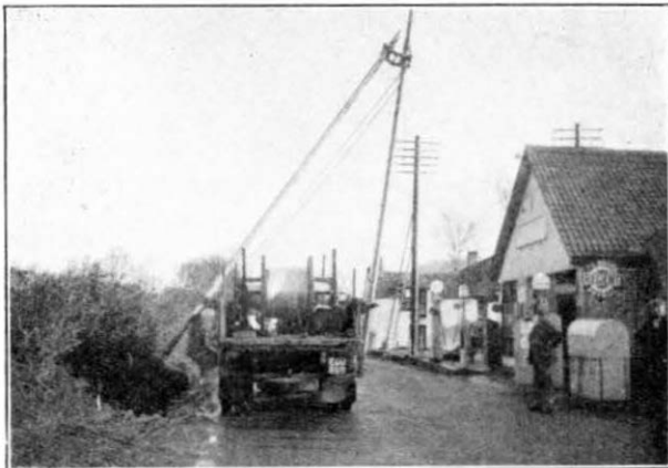
FIG. 1.—THE LADDER DERRICK.
