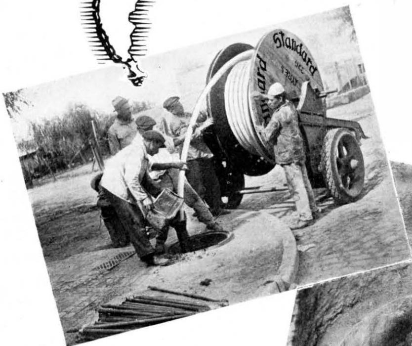
Lead-covered Cable about to be drawn into duct.
