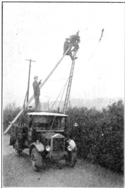
FIG. 10.—DERRICK USED TO ERECT AERIAL CABLE.
