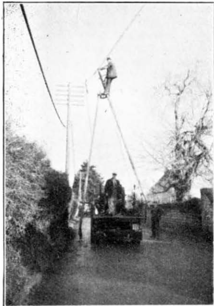
FIG. 7.—DERRICK USED IN VERTICAL POSITION.
