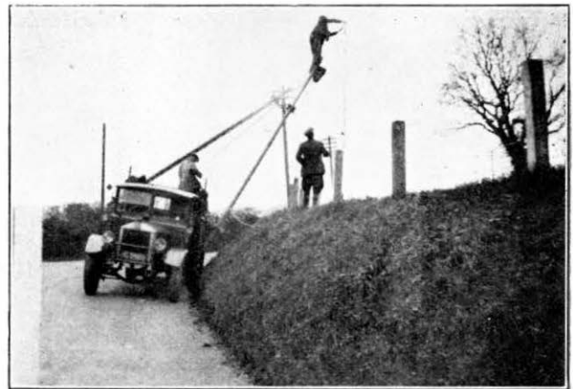
FIG. 6.—DERRICK USED WITH MAXIMUM OVERHANG.
