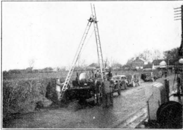
FIG. 4.—ERECTOR OF DERRICK.
