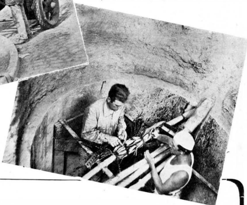
Joining operations in progress.
