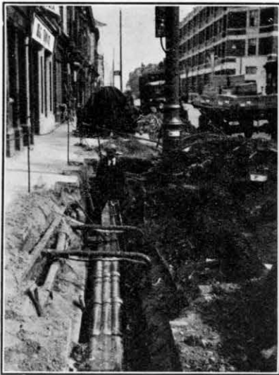
FIG. 2.—COMPLETION OF REPAIRS TO DUCT.
