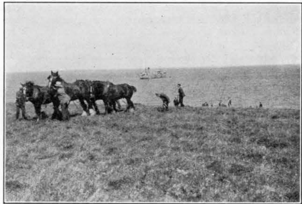
FIG. 1.—HAULING THE CABLE TO THE HEADLAND.
