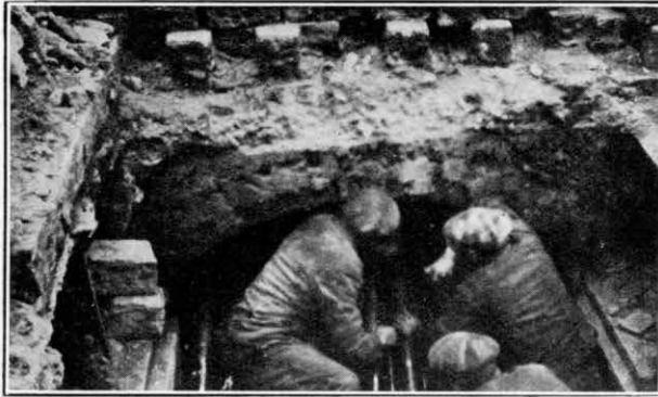
FIG. 1.—LAYING THE LAST PIPE.
