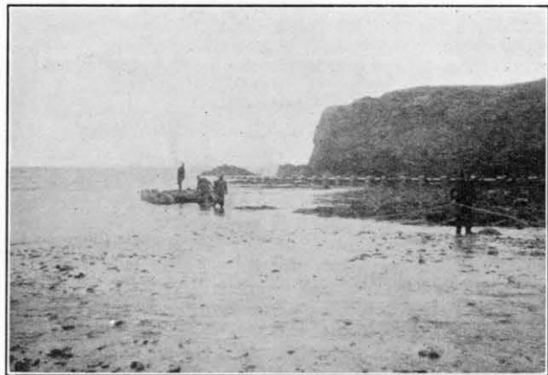
FIG. 2.—LANDING THE CABLE FROM THE RAFT.
