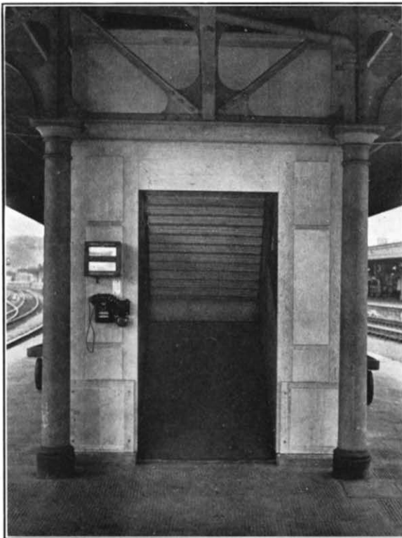
FIG. 4.—DISCHARGE ON RAILWAY PLATFORM FROM TWIN-BAND RISER.
