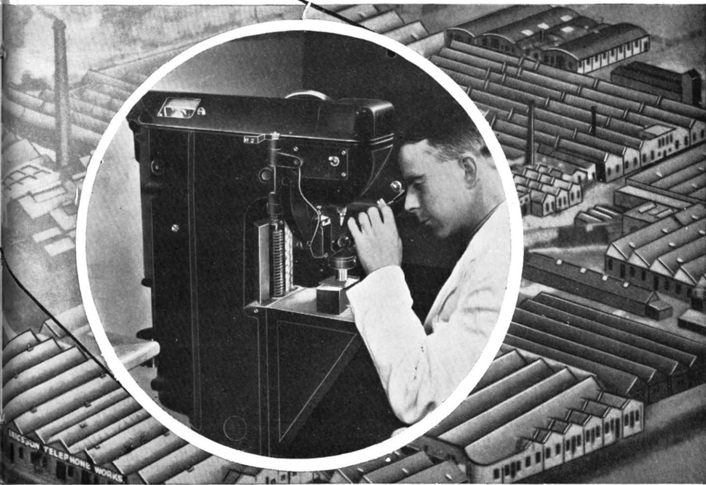
2. Testing the hardness of materials.
