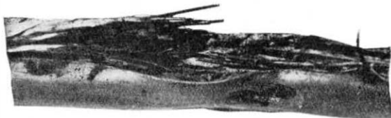
FIG. 7.—CABLE FAULT CAUSED BY LIGHTNING.
