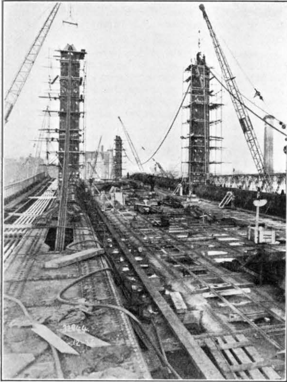
FIG. 1.—VIEW OF BRIDGE UNDER CONSTRUCTION.
