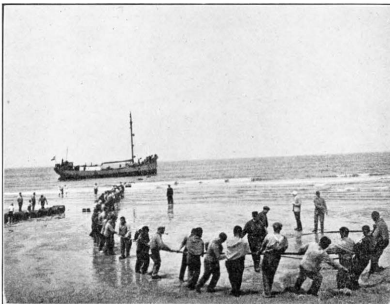
FIG. 2.—LANDING THE SHORE END AT DOMBURG.
