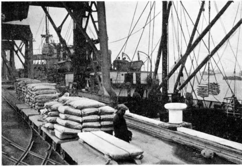
FIG. 9.—LOADING CEMENT IN PAPER BAGS.
