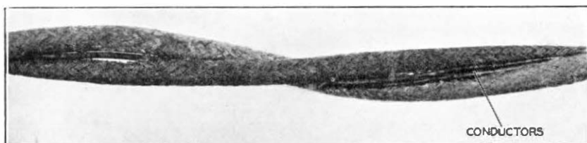
FIG. 5.—INSULATED WIRES DAMAGED BY LIGHTNING.
