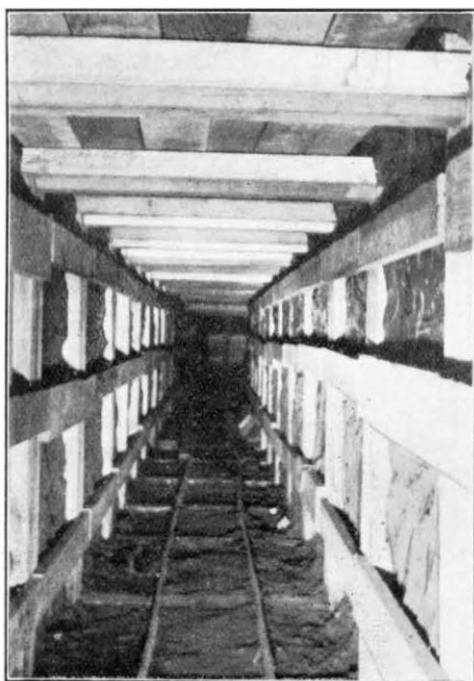
FIG. 1.—HEADING FOR 99-WAY DUCT ROUTE.
