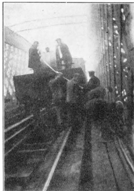
FIG. 2.—CABLE LAYING OPERATIONS.
