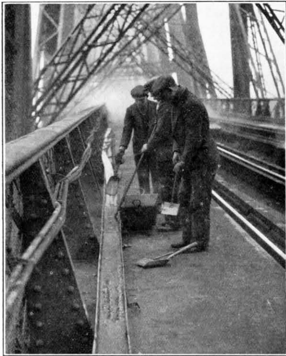
FIG. 4.—FILLING THE TROUGH WITH COMPOUND.
