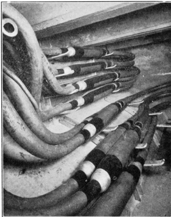
FIG. 5.—COMPLETED JOINTS IN MANHOLE OUTSIDE BRETENHAM HOUSE.
