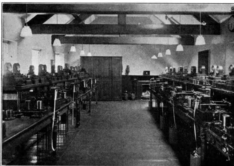
FIG. 2.—OLD REPEATERS AT THE LLANFAIR STATION.
