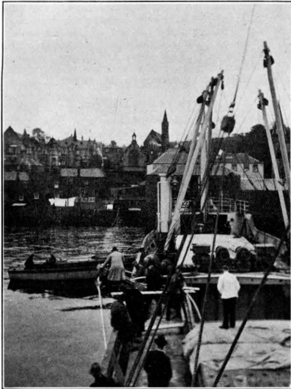
FIG. 2. PULLING THE SHORE-END OUT OF THE HOLD.
