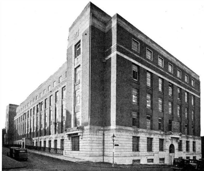
Telephone House, Birmingham
