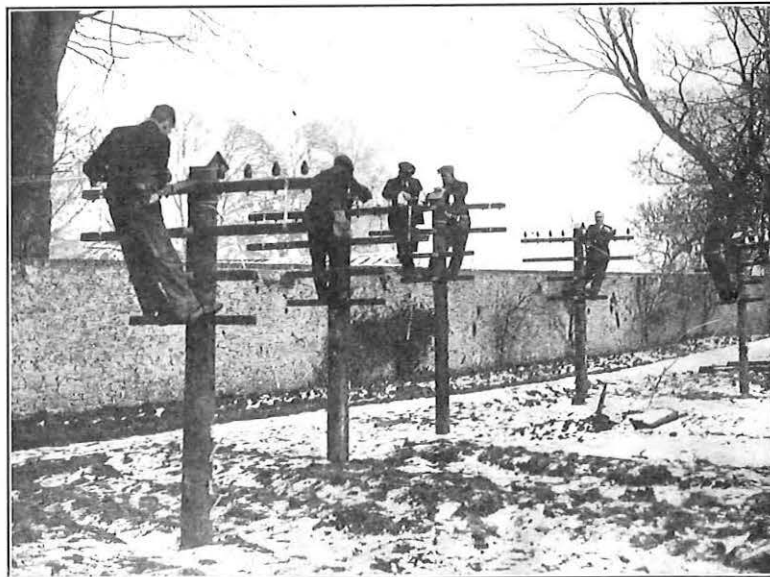
FIG. 5.—EXTERNAL WORK ON SHORT POLES.
