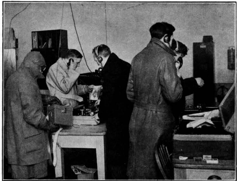
FIG. 5.—LINEMEN'S ROOM IN USE FOR PICTURE TRANSMISSION.
