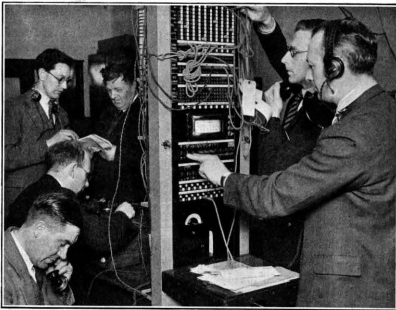
FIG. 1.—SETTING UP ADDITIONAL CIRCUITS AT KING'S LYNN.
