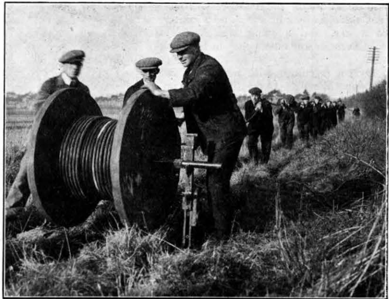
FIG. 3.—HAULING TEMPORARY CABLE BY HAND.
