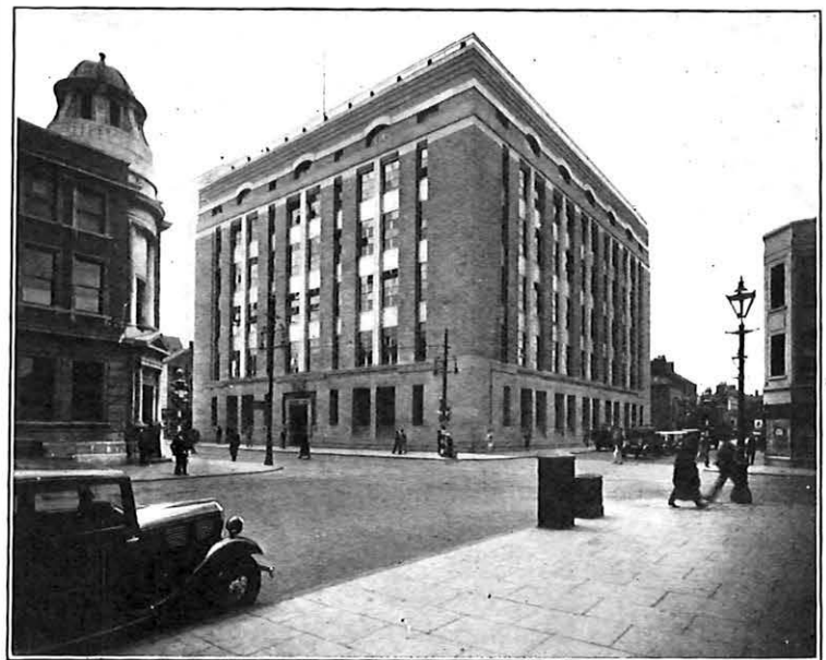
FIG. 4.—TELEPHONE HOUSE, BELFAST.
