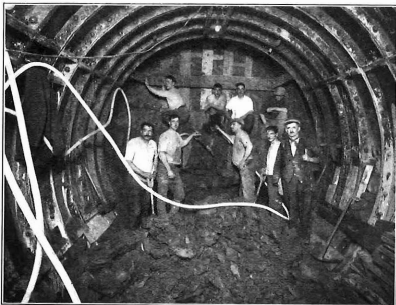
FIG. 15.—NEW L.C.C. SUBWAY UNDER CONSTRUCTION.
