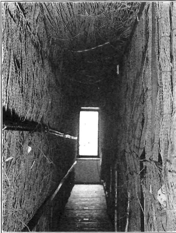
FIG. 3.—M.D.F., OLD BELFAST CENTRAL EXCHANGE.
