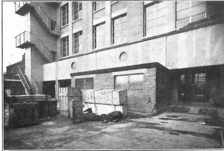
FIG. 10.—EXTERIOR OF CABLE CHAMBER.
