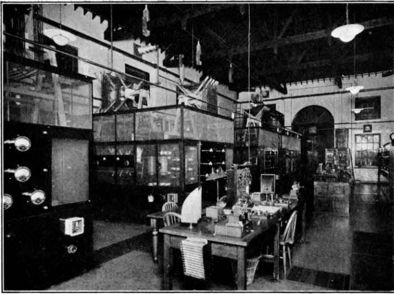
FIG. 2.—MAIN TRANSMITTING ROOM.
