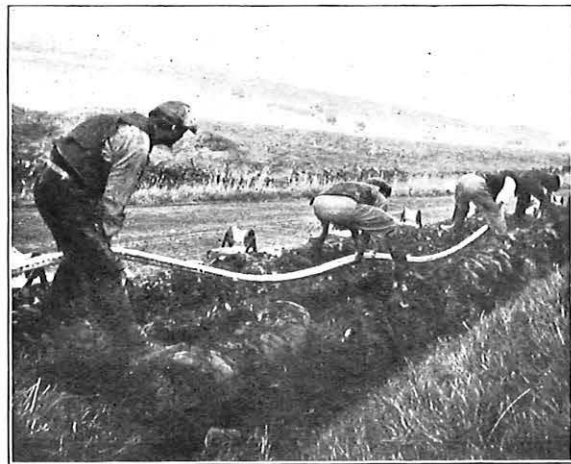
FIG. 4.—LIFTING THE CABLE INTO THE TRENCH.
