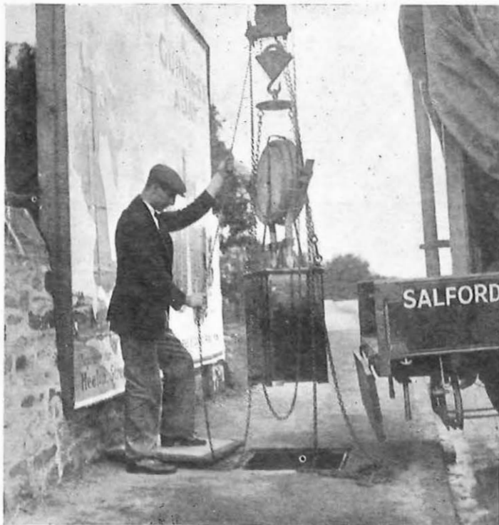
G.E.C. loading coils being lowered into a manhole near Lancaster, 1934.
