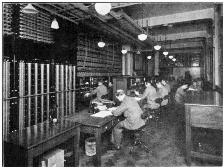
FIG. 4.—TEST DESK AND MAIN FRAME, AUTO EXCHANGE.
