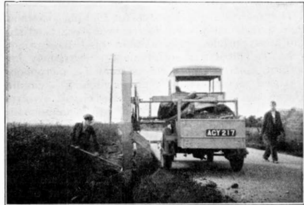
FIG. 14.—TRENCH EXCAVATING MACHINE.
