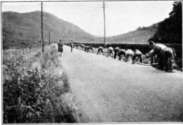
FIG. 10.—CABLING IN PROGRESS NEAR BEATTOCK.
