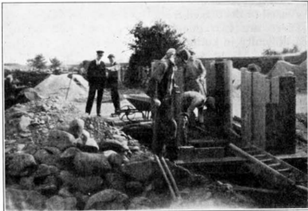
FIG. 12.—NATURE OF SUB-SOIL AT MANHOLE EXCAVATIONS.
