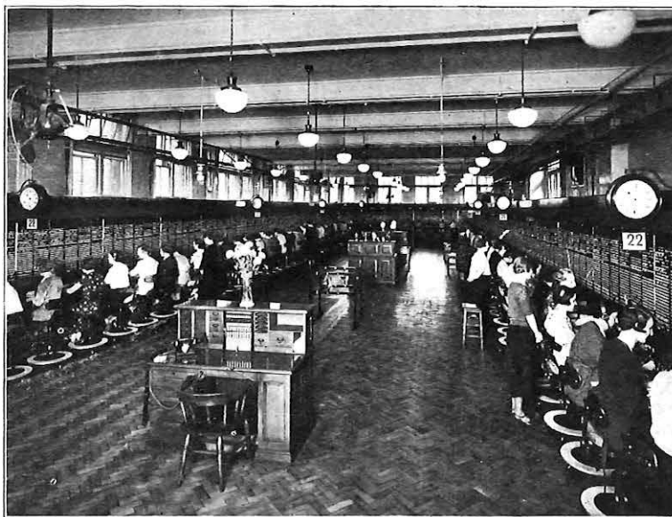
FIG. 6.—THE NEW MAIN TRUNK SWITCHROOM.
