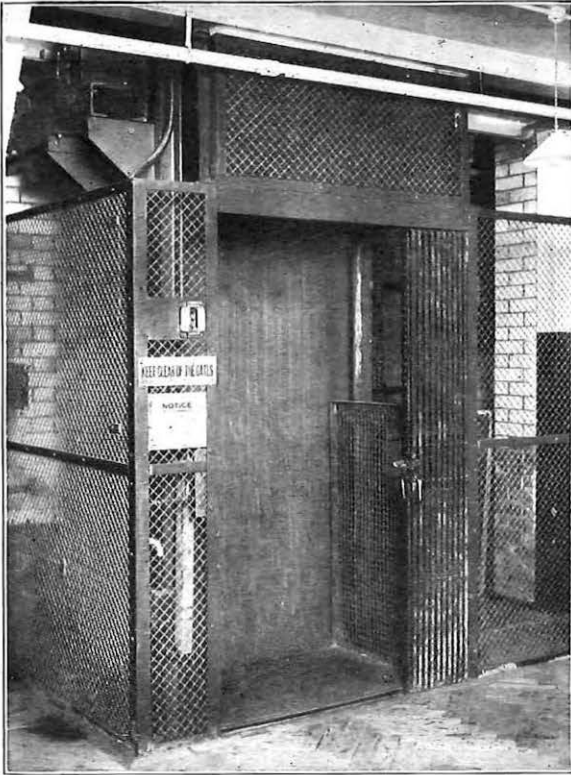
FIG. 4.—VIEW OF PAVEMENT LEVEL ENTRANCE.
