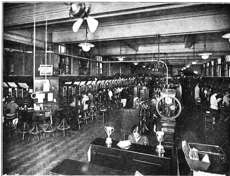
FIG. 5.—THE OLD TRUNK SWITCHROOM.
