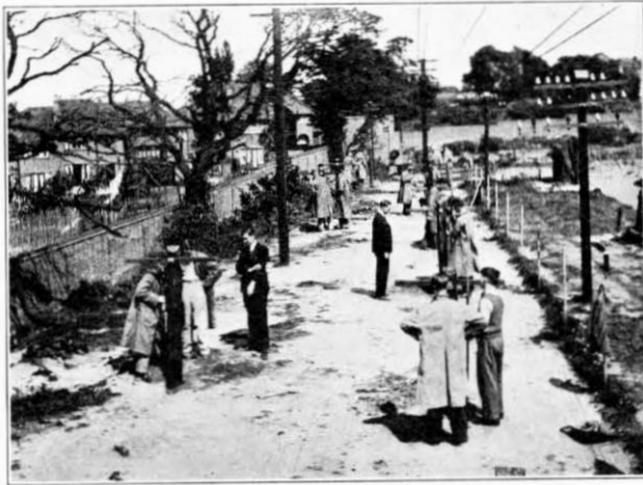
FIG. 2.—VIEW OF CONSTRUCTION PARK.
